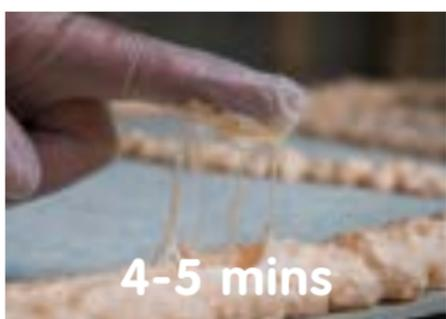
5. For bonding HardieBacker® board to any surface: wait until the adhesive is partially cured (approx. 4-5 minutes) for optimal grab. This can easily be checked:
