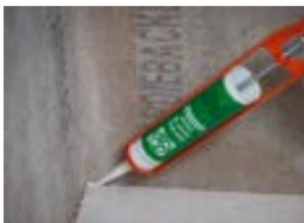
7. Leave a 3 mm perimeter gap and fill with a good quality bathroom sealant.
