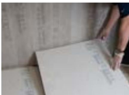
8. Install subsequent boards in moderate contact using a brick bond pattern.
