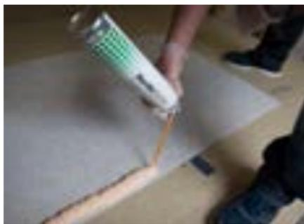
3. Lay the board flat. For adequate coverage, ensure a 25 mm bead of foam is applied 25 mm from the perimeter of the board and the area inside in a zigzag pattern.
