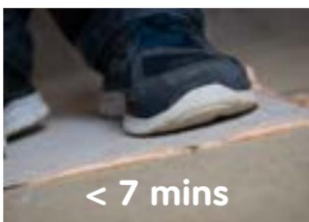
6. Bond the HardieBacker® to the wall or floor within a maximum of 7 minutes. The HardieBacker® should be pressed to the surface with a sliding action. This helps spread the foam improving the bond. Hold for 30-60 seconds. For floor applications, walking on the boards will assist greatly. Ensure all edges of the board are firmly bonded and flat. Lipping to adjacent boards should be kept to a minimum.
