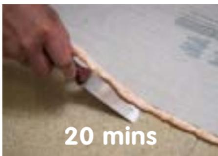
9. Excess HardieFoam™ should be removed from the surrounding area after around 20 mins, before fully cured, using a suitable pallet knife.
