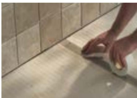
10. HardieBacker® joints should be taped with HardieTape™ and then filled with tile adhesive to produce a 150 mm wide feathered joint.
